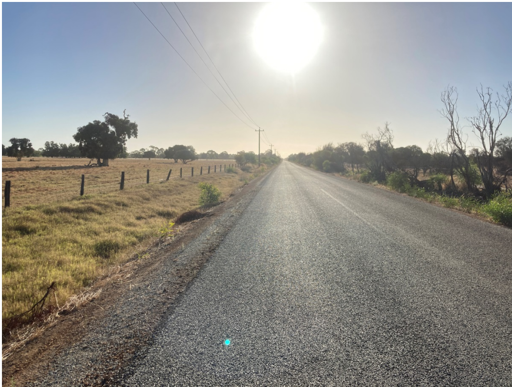
Photograph 1: Timaru Road 100 m East of Brand Hwy facing west
