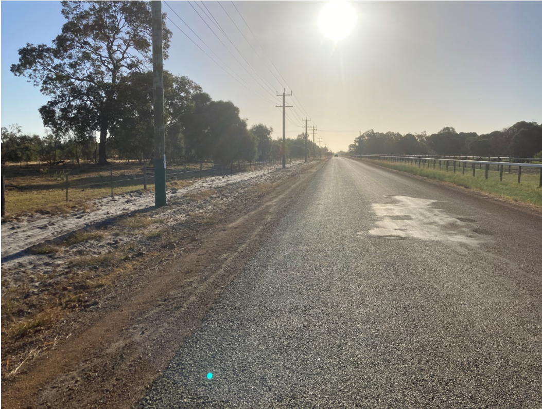
Photograph 3: Timaru Road 1000 m East of Brand Hwy facing west
